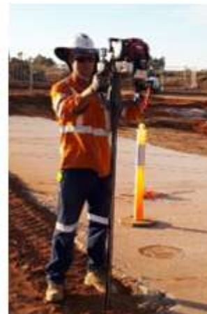
Photo 6 Preferred method for the installation of star pickets, (motorised driver)
