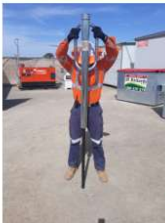
Photo 5 Incorrect method of using Star Picket Driver. Hands must not be positioned about shoulder height.
